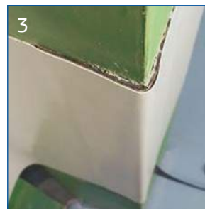
3 Fit wall covering and pull tight and flat around external corners.
