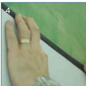
4 Use either QT100 or QT200, depending on thickness of wall covering, to allow for joints to be made between two coverings.
