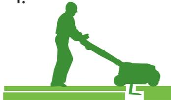
Strip turf removing all the grass down by an average thickness of 50mm with a motorised turf cutter or a sharp spade. At this stage you can also lay a lean mix concrete around the perimeter for fixing the grass to if you desire.
