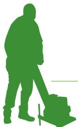
Set and finish perimeter heights at approx. 15mm below the edge system. Wet down the area and compact the sand using either a plank and sledge hammer or a motorised plate compactor.
